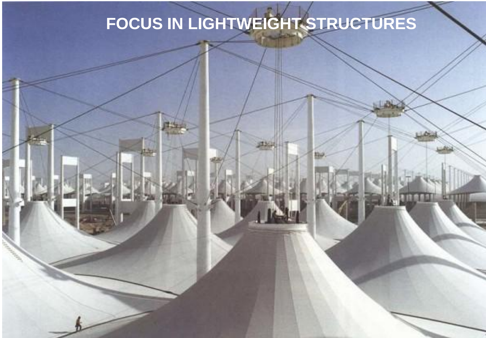
HAJ TERMINAL JEDDAH AIRPORT SAUDI ARABIA - HORST BERGER
