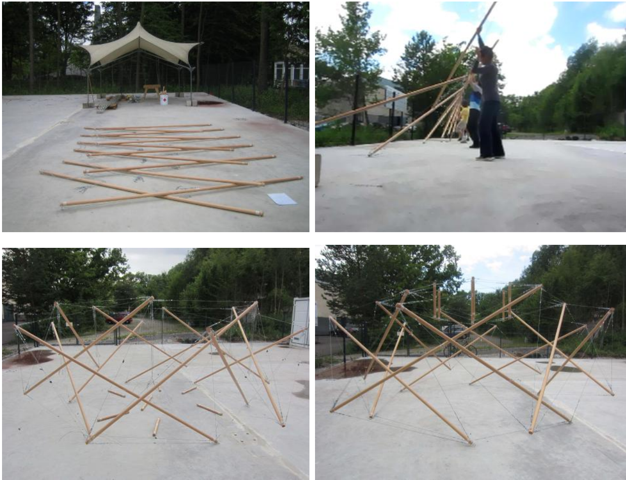
Fig. 01 Tensegrity prototype assembly - ESC_1:10
